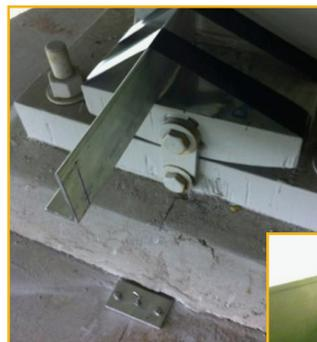
Displacement gages are mounted on the rocker bearings to monitor movement away from the supports as the bridge expands and contracts in response to changes of up to 70°C
